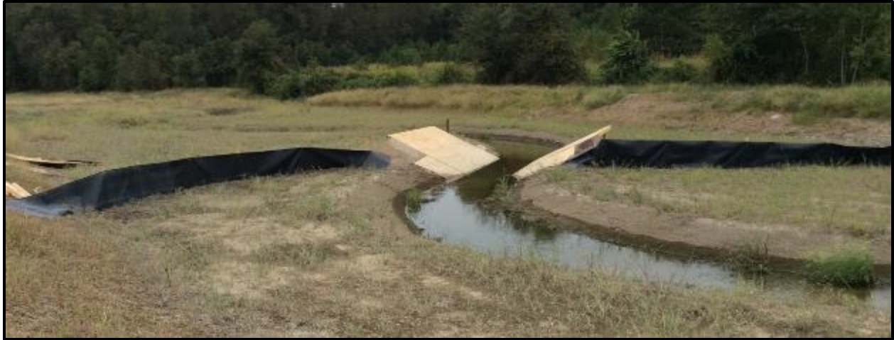
Figure 8. Image of the trapezoidal wooden section and the floodplain curtain at CLMD during construction
